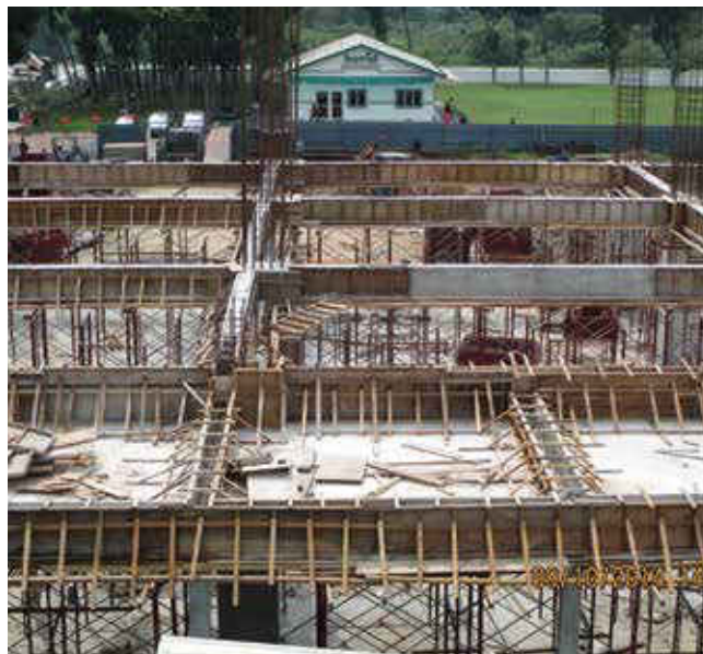
Construction Site of Plant A
